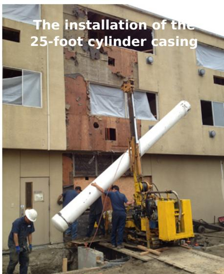
The installation of the 25-foot cylinder casing
